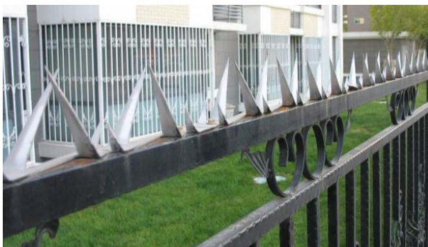
Bayonet mount spikes used on fence topping
