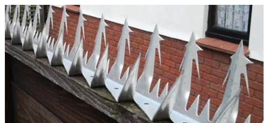
Wall spikes used on wood fence
